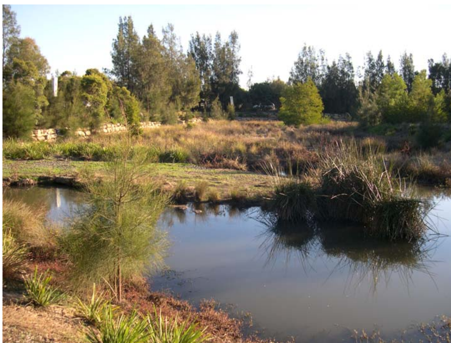
Figure 2. A free water surface constructed wetland (FWS CW) for stormwater runoff in Woodcroft Estate near Sydney, NWS, Australia. Photograph taken by the author.
